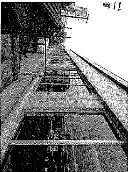
Laboratory analysis identified the pink paint finish on the exterior concrete walls to be lead containing.
