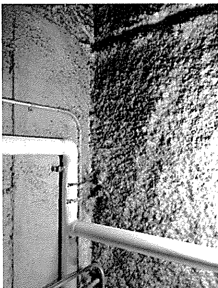
Fulcrum observed a white fluffy sprayed on fireproofing material in the upper mechanical room.
